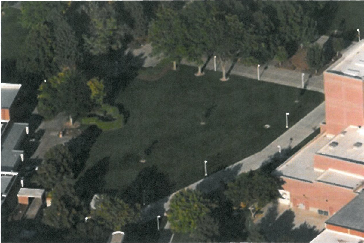
Fig. 3: Aerial view looking north/northeast between Gymnasium (left) and Fine Arts Building
