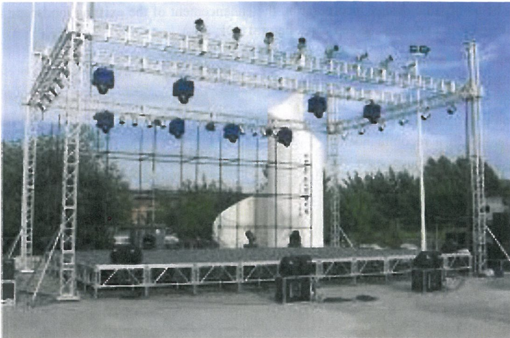
Fig. 25. Example of amphitheater lighting system
